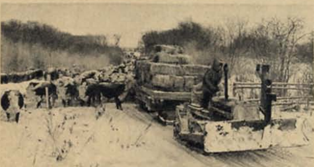
BULLDOZER PLOWS TRAIL. HAULS SLED
